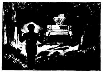
② The tank commander must dismount and precede the tank on foot, directing the driver into the assembly position by dimmed light signals.
