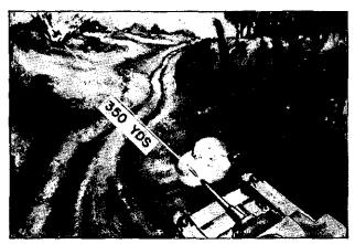
1 Do not fire at antitank gun with 37-mm tank gun at close range.
